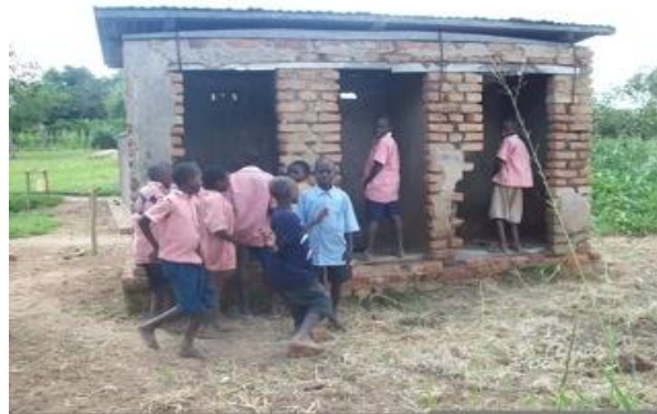
This is the latrine we are replacing
